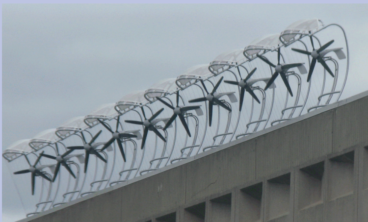
Ten 1-kilowatt micro-wind turbines were placed on Becton Center in the spring of 2009.
