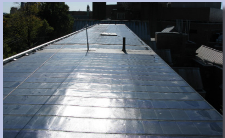
Thin-film solar modules were installed on Yale's Swing dorm in the summer of 2009.
