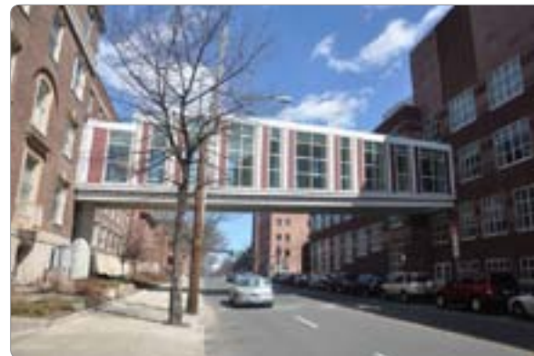
Bridge over Congress Ave.
