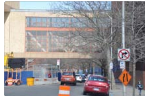
Bridge over York St.
