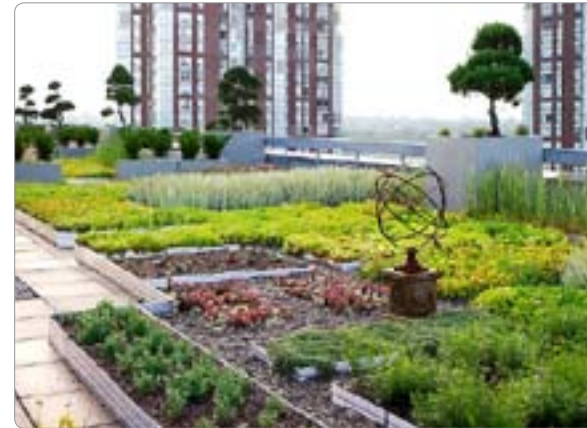
ESRI Headquarters Green Roof
