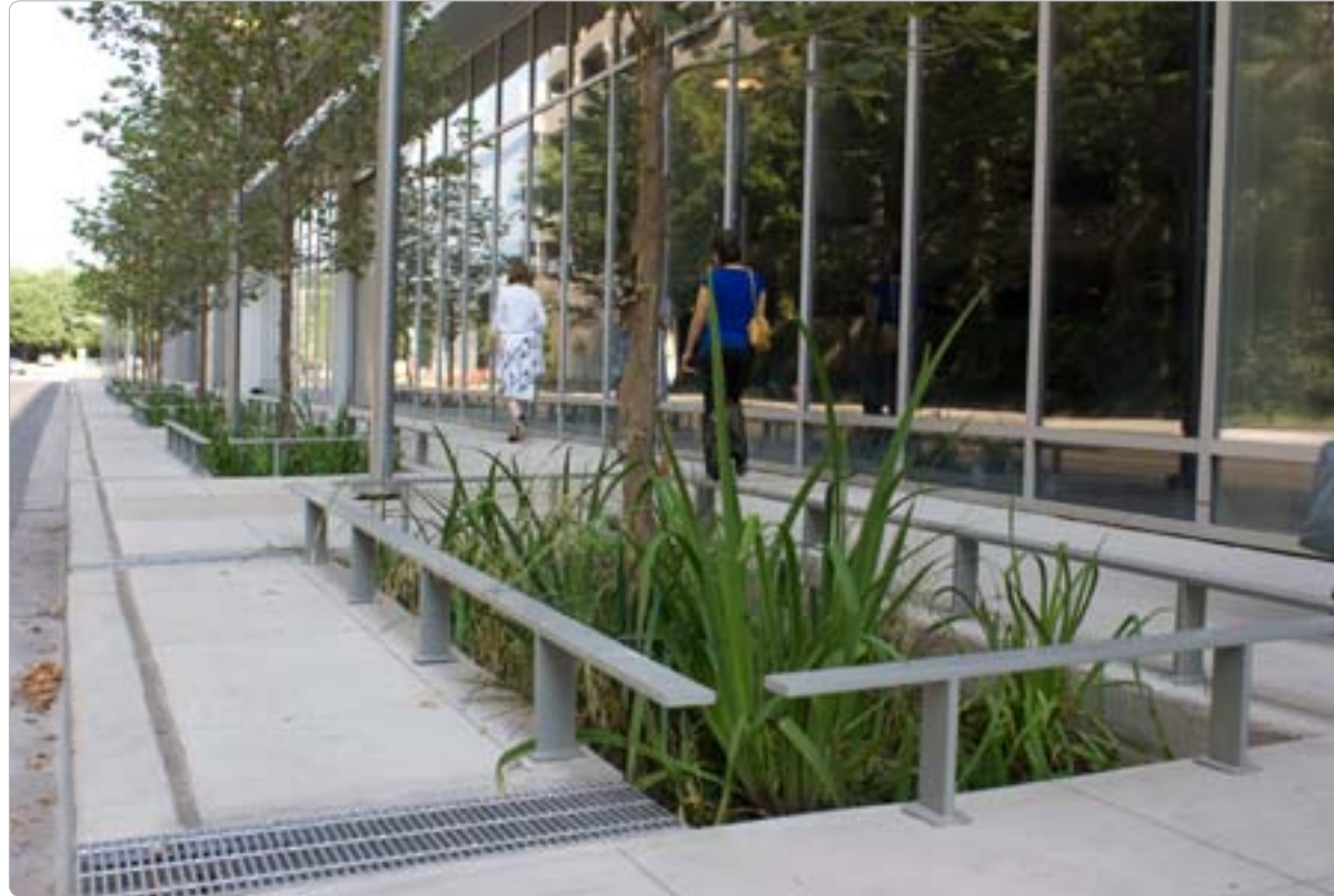
Low Maintenance Storm Water Planters, Rush University Medical Center
