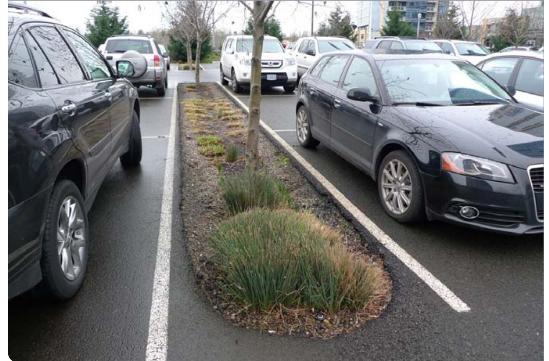
Planted Swale, OHSU Portland
