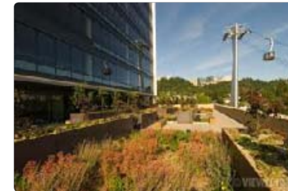
OHSU Roof Garden
